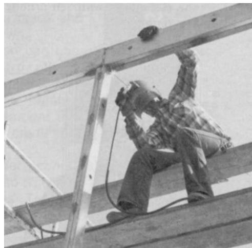
An overall view, from the second floor, shows the two-story wall panels that have been fabricated from Super-C steel studs. The worker on the scaffold is welding perimeter joists to the tops of the wall panels.
