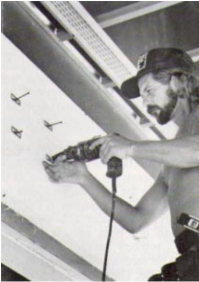
Mechanical fasteners provide exceptional strength for attaching EIFS to gypsum board, and allows the foam to be attached quickly.
