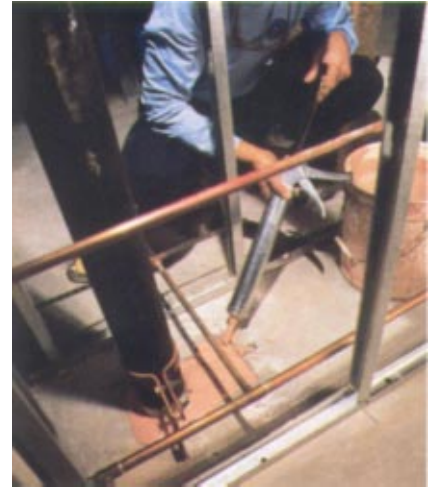
The compound is mixed on-site with water (left photo), then it is caulked over the insulation (two right photos).
