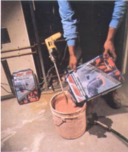
The compound is mixed on-site with water (left photo), then it is caulked over the insulation (two right photos).
