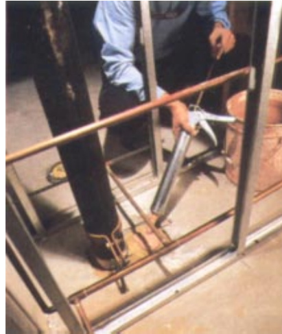
The compound is mixed on-site with water (left photo), then it is caulked over the insulation (two right photos).
