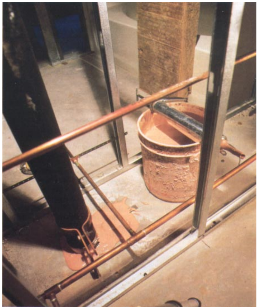
The compound dries to a pink color, which can be easily identified by fire code inspectors.
