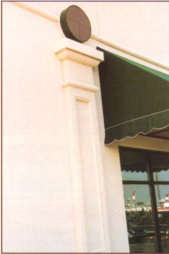
*The project involved extensive use of expanded polystyrene insulation boards, which were cut into ornamental shapes, columns and cornice details.*
