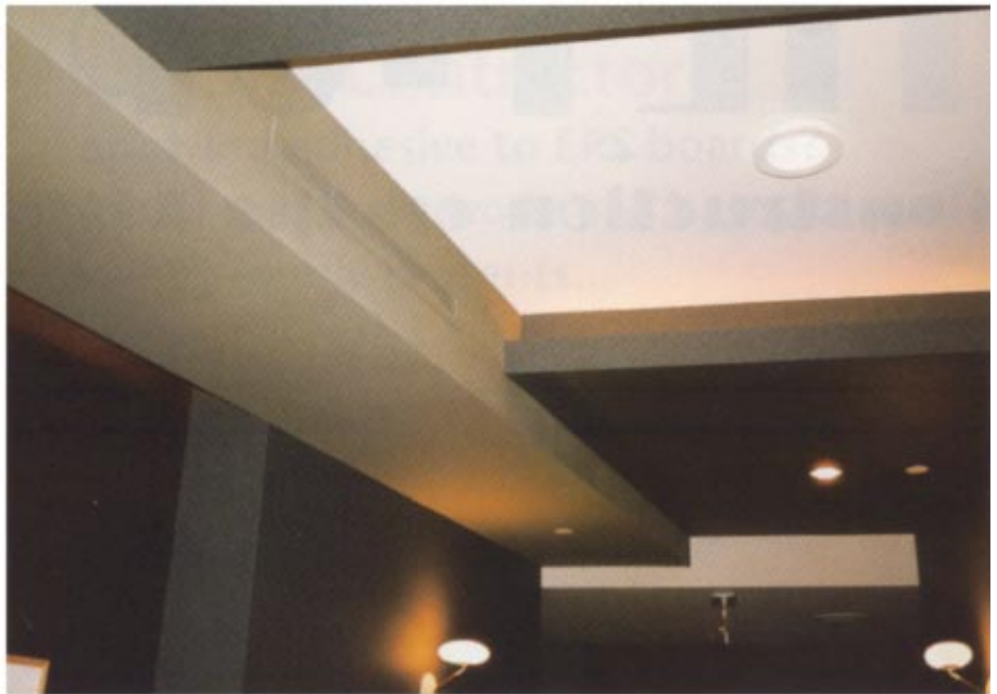
The “nouveau industrial” design combined exposed decks with recessed wall spaces for displaying artwork, curved soffits and finished drywall to the deck.
