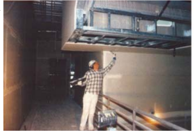
In critical lighting areas, flat paints applied over light textures tend to reduce joint photographing.
