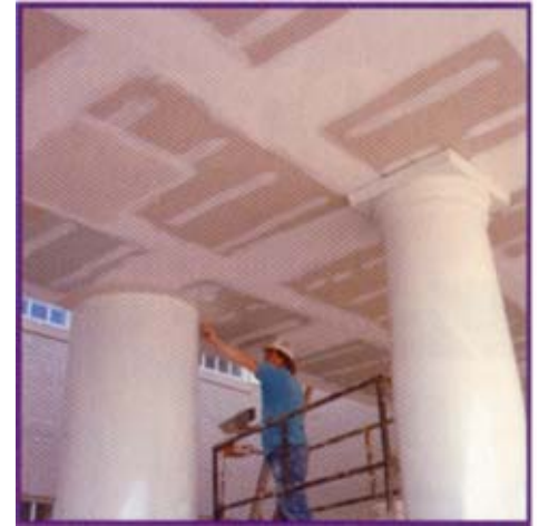
Lighting is critical, especially when trying to achieve a Level 4 or Level 5 finish.
