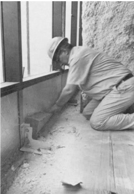
Effective fire protection materials, such as Thermafiber Safing, left, and Thermafiber Curtain Wall Insulation, right, as installed in Sears Tower, Chicago, virtually eliminate fire spread as described in new movie.
