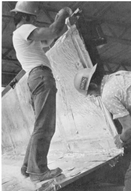
Effective fire protection materials, such as Thermafiber Safing, left, and Thermafiber Curtain Wall Insulation, right, as installed in Sears Tower, Chicago, virtually eliminate fire spread as described in new movie.
