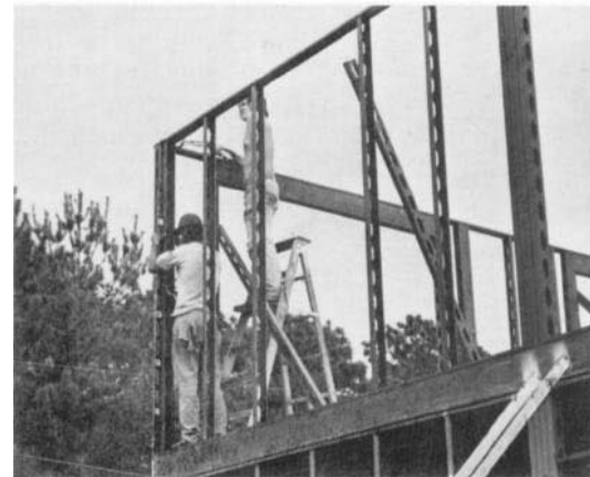
Each panel (above) is plumbed and temporarily braced. Below, the floor of roof framing is set on the load bearing steel frame wall.
