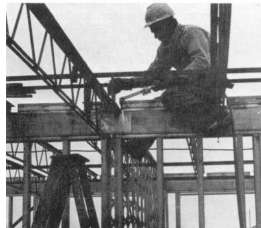
Each panel (above) is plumbed and temporarily braced. Below, the floor of roof framing is set on the load bearing steel frame wall.
