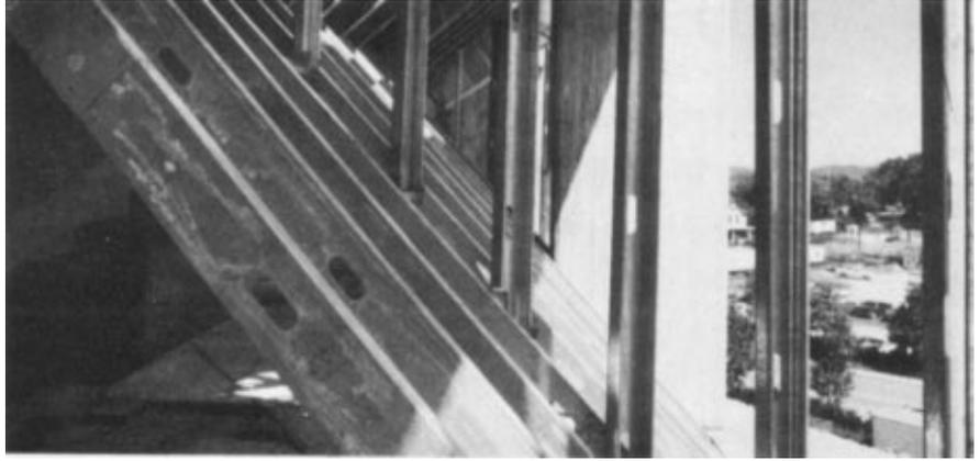
Light gage steel is useful for interior partitioning, but load bearing steel is just as important and not a great deal more difficult to install.
