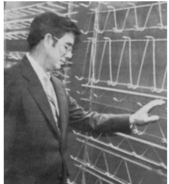
Bostwick's Gris Hurlbert inspects steel work used in concrete wall assemblies.
