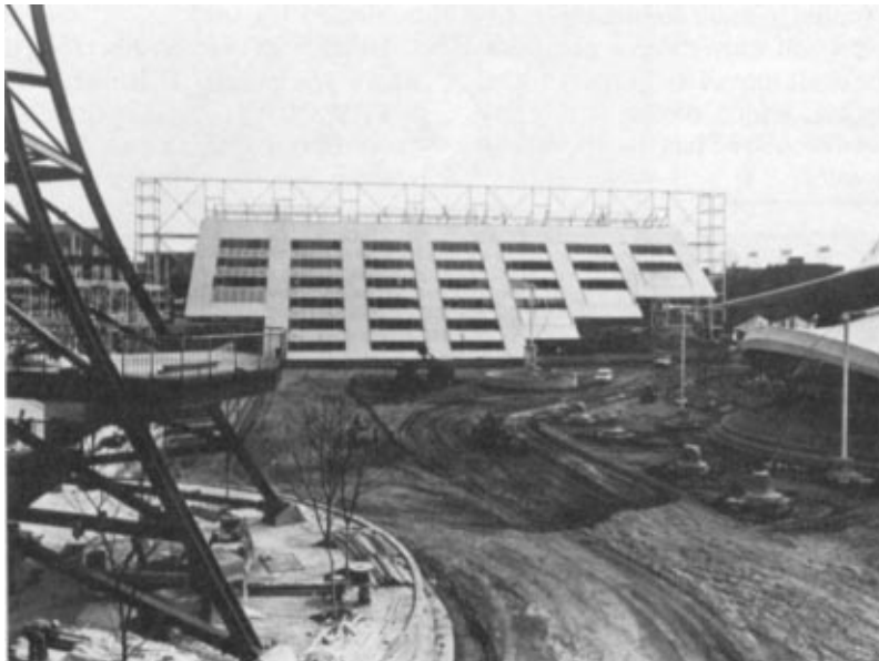
Both the Sunsphere (left foreground) and the US. Pavilion (background) have steel studs.
