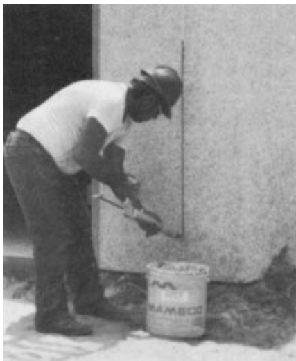
The applicator is shown putting sealant into the joint (left) and then tooling it off (right)
