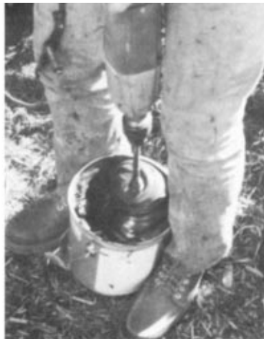
Power mixing of a 2-component sealant is efficient and assures a good mix.
