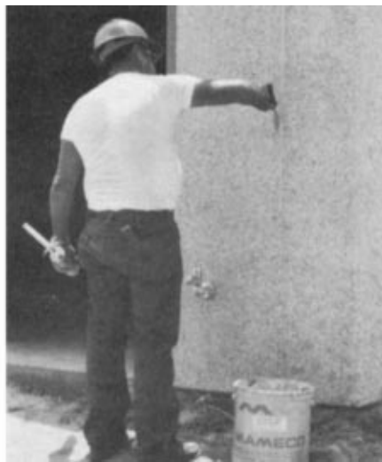
The applicator is shown putting sealant into the joint (left) and then tooling it off (right)
