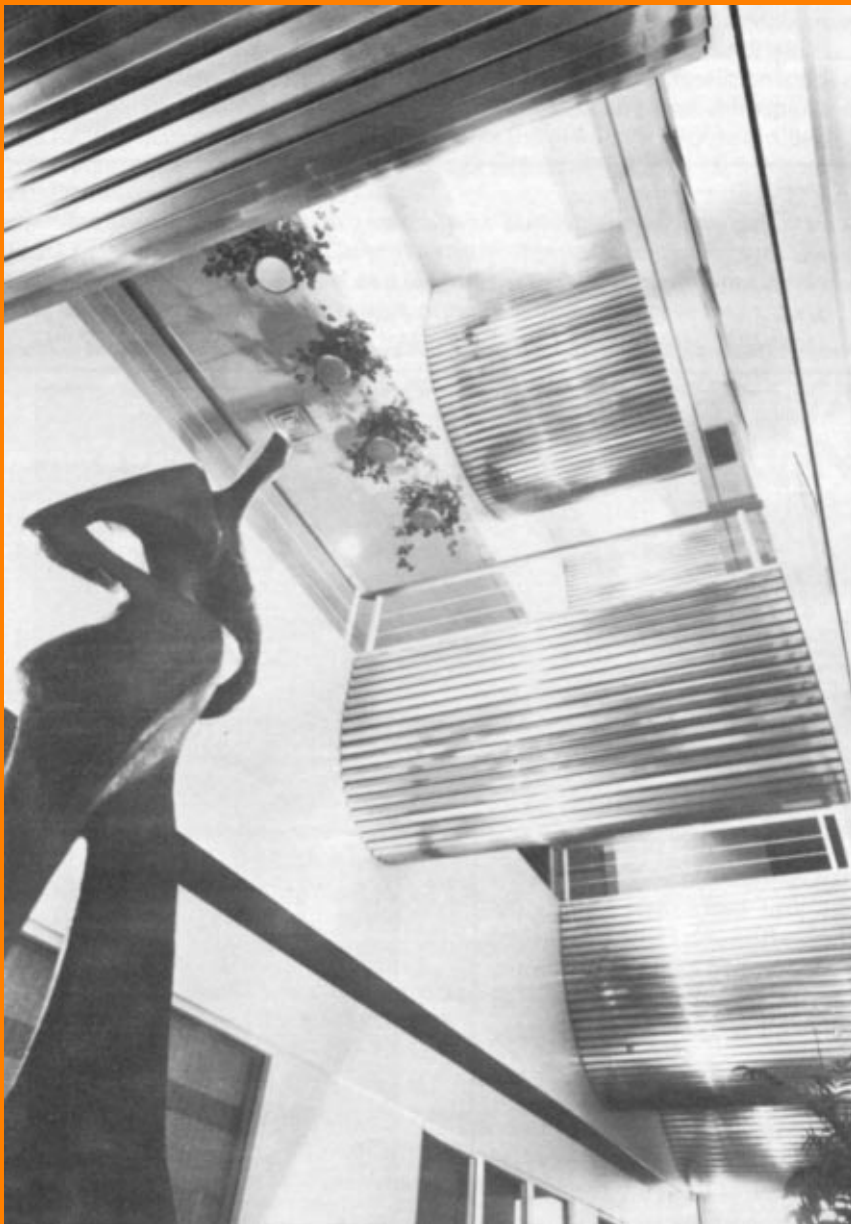
Linear ceilings can be formed easily to both concave and convex curves.
