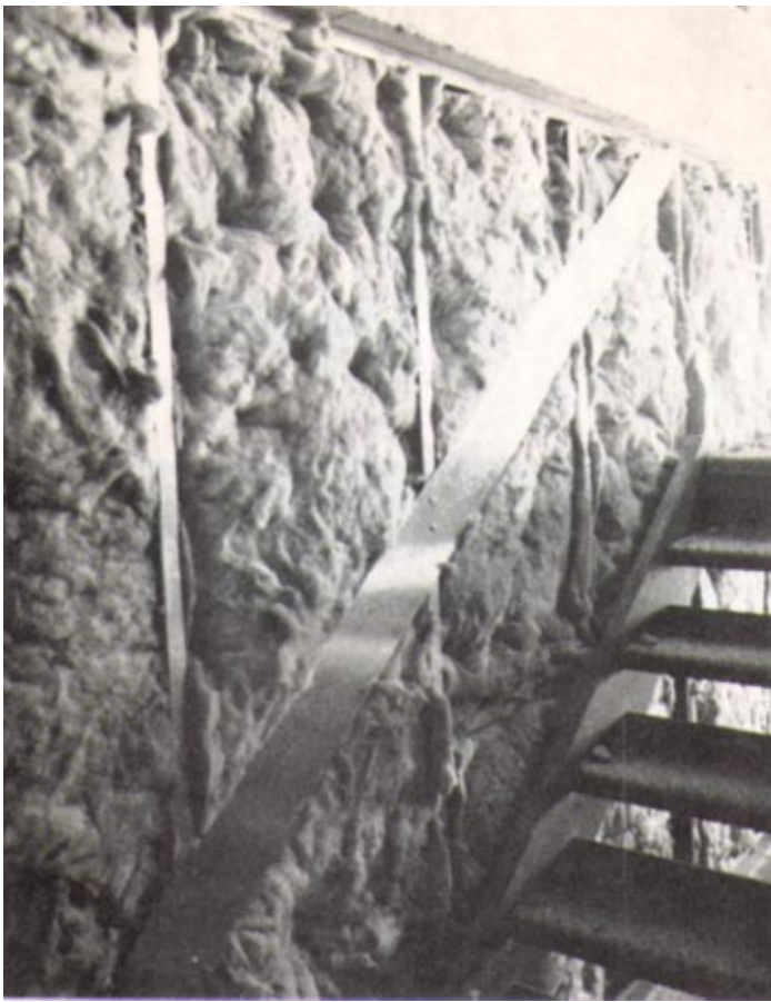
8" x 20" ga. continuous metal stripping attached to each stud prior to installation of gypsum board.
