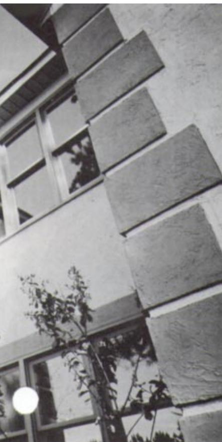
terior basecoat (a ready-to-mix latex-fortified Portland cement mortar) which is applied over the tape and forced into the joints. Treated joints cure for a minimum of 24 hours. Next, the same basecoat is applied over the entire board area. After another 24-hour cure time, exterior finish is troweled on to provide desired texture. The exterior finish features a 100 percent acrylic polymer elastomeric coating to accommodate thermal expansion and contraction without cracking or delamination.
