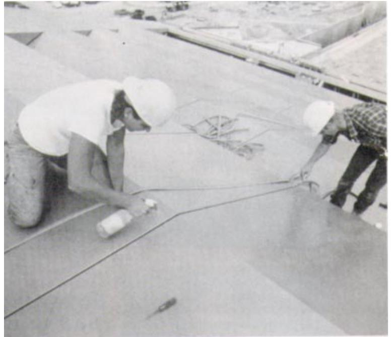
*Placement of a silicone gasket at the panel joints was the final step in installation of the panels. A lubricant was then sprayed on the gutter and a gasket is placed over it before the gasket was pressed into place with a hand tool.*
