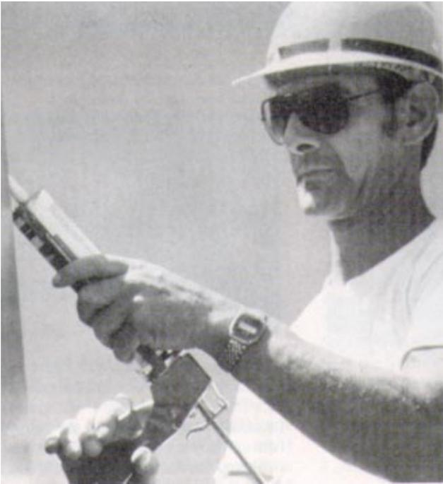
*Panels were engaged to adjoining panels with a male/female fit followed by a silicone sealant, applied to the joint.*
