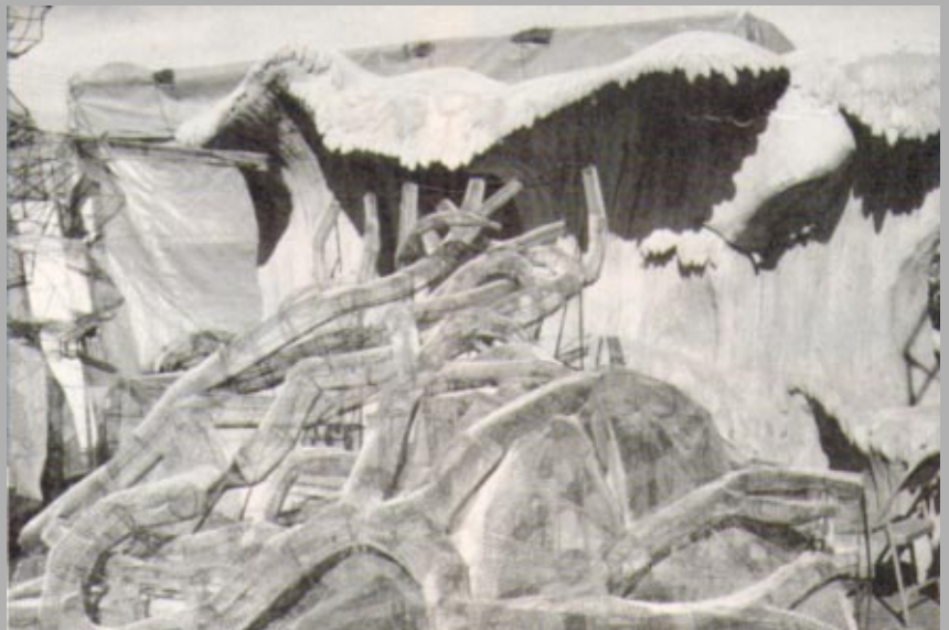
Finished cage in foreground awaits transfer to Splash Mountain job site for welding to the steel structure skeleton. Plaster sculptured section in background will not be used. It was made only for testing and experimental purposes, one of the many trial runs necessary before final construction decisions could be made.
