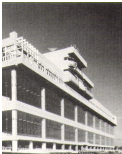
The grandstand of the $90 million Remington Park race track in Oklahoma City required installation of 133,000 square feet of exterior insulating finish systems (EIFS).
