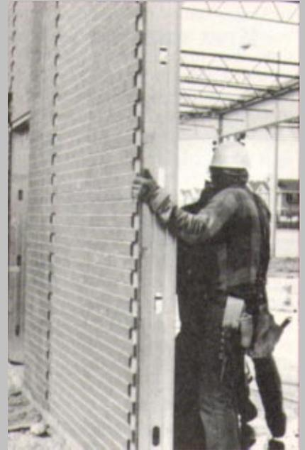
*Thin brick panels using Durock Exterior Cement Boards were set on footings for the Hungry Fox Restaurant.*
