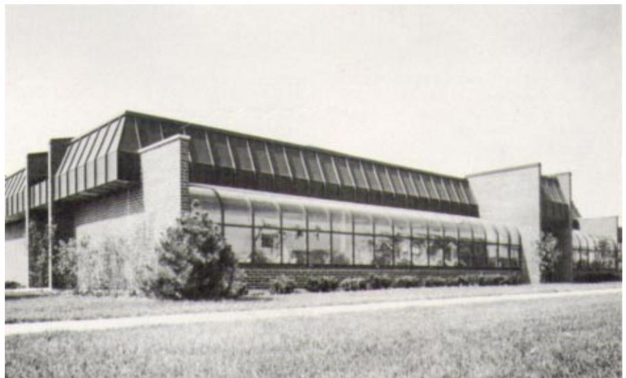
*The Hungry Fox Restaurant in Wheeling, Illinois was one of the first to use prefabricated panels of Durock Exterior Cement Board with thin brick veneer.*
