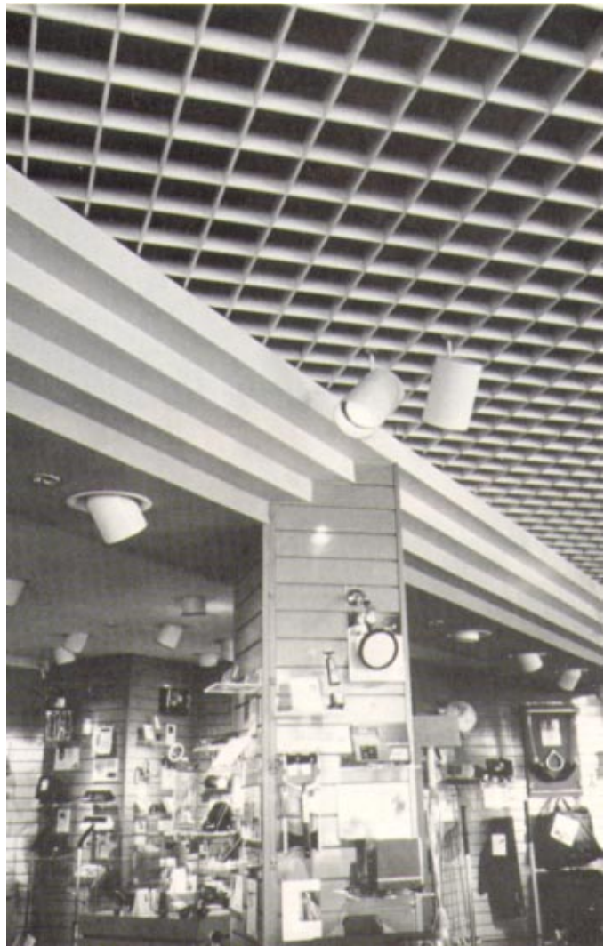
This photo shows MAGNAGRID specialty metal open-cell ceiling system from Alcan Building Products.
