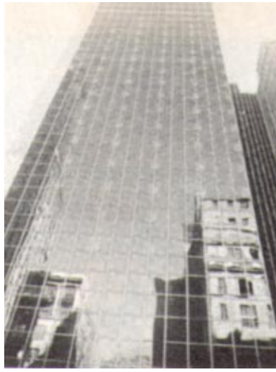
Glass curtainwall by Kawneer on Tower 49, New York, New York. Architect: Skidmore, Owens & Merrill. Contractor: Tishman Construction Corporation.
