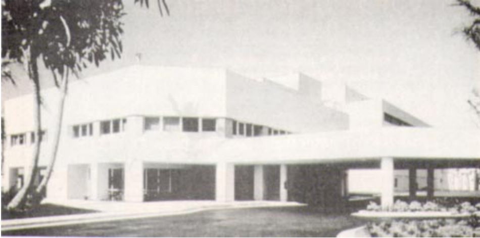
Insulation/stucco wall by Insul-Crete/Dow Chemical on the Cape Coral Hospital, Cape Coral, Florida. Architect: Hanson, Lind, Meyer. Contractor: Mellon-Stuart (AGC).
