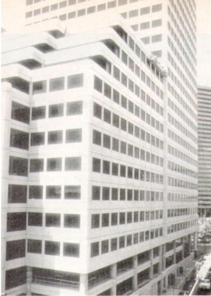
Precast concrete panel by Bluegrass Art Cast on Atrium Two, Cincinnati, Ohio Architect: Skidmore, Owings & Merrill. Contractor: Huber, Hunt & Nichols (AGC).
