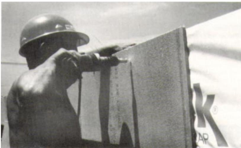
1. Installation begins with the application of a required water barrier such as Tyvek Housewrap, as seen here, or No. 15 asphalt felt. Then, panels are attached horizontally or vertically to the studs using screws spaced a maximum of 8-in. o.c. (hot-dipped galvanized roofing nails can also be used to attach the board).
