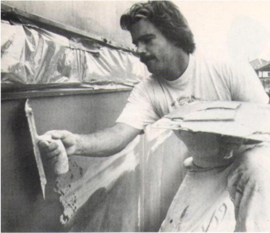
*3. Then, the ready-to-mix, portland cement exterior basecoat is applied over the entire board area at a minimum thickness of 1/16-in. and allowed to cure for at least 24 hours.*
