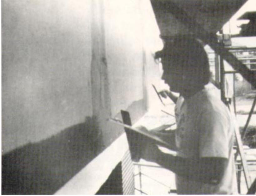
2. Next, tape is applied over the joints and the exterior basecoat is forced through the tape to completely fill and level the joints. The treated joints are allowed to cure for at least 24 hours.
