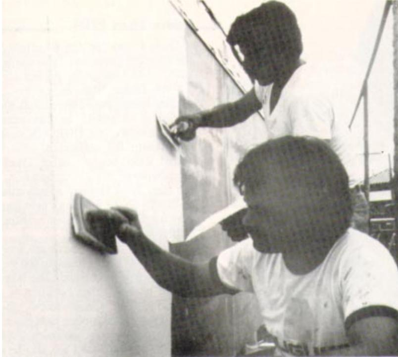
*4. Finally, the exterior finish is applied in a minimum 1/16-in., maximum 3/16-in. thickness using conventional tools and techniques to achieve a variety of stucco looks. Here, the finish is being troweled on and then floated to achieve the desired look.*
