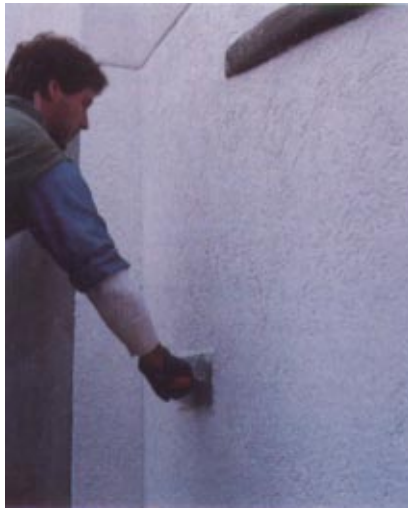
To obtain high build texture and color uniformity in one step, apply a trowel applied acrylic finish coating, commonly referred to as "synthetic stucco."
