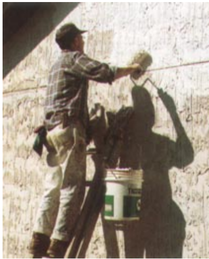
A 100% acrylic coating is ideal for obtaining a uniform, durable finish for the stucco surface.
