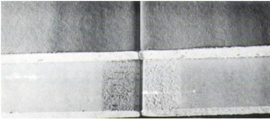
*Fig 1: Comparison of HA taper to regular gypsum board (on top).*
