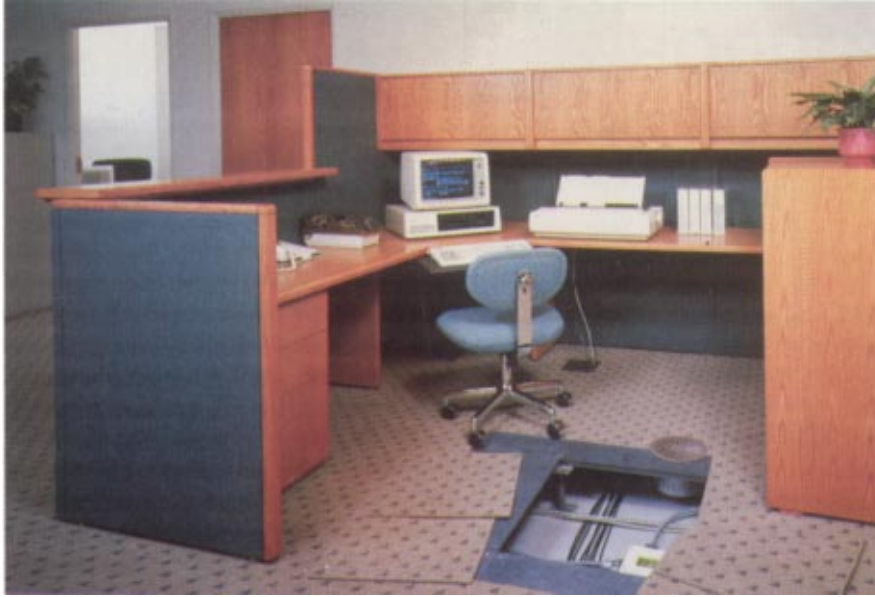
Air distribution control plenum system provides upward air supply.
