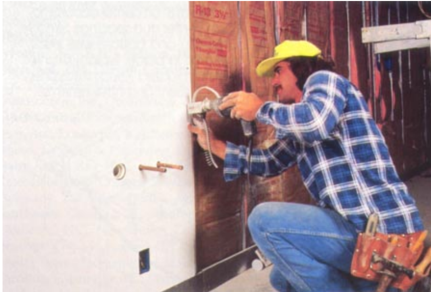
Fire-resistant steel studs and track are installed in each Checkers building.
