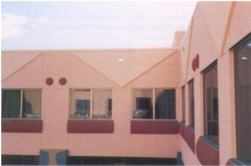
*The finish provides a "waterslide" effect to repel water quickly and thereby minimize harmful buildup of mildew on the building's surface.*
