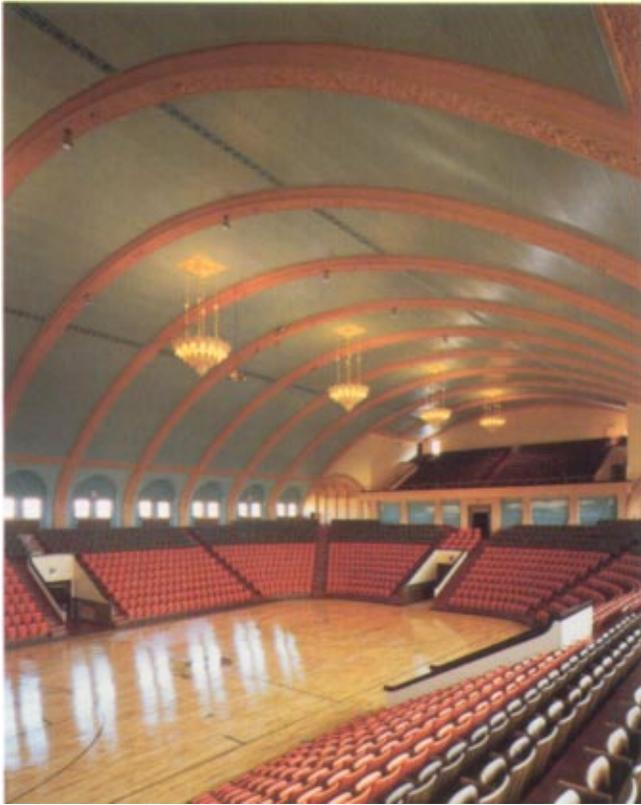
*The above installation features 6 inches wide Vista panels with flush filler strips. The panels are perforated providing a more acoustically pleasing interior.*
