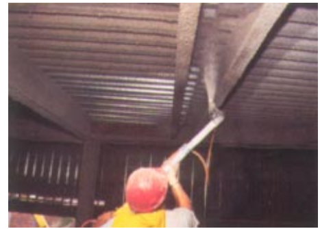
For the hotel, casino and family entertainment areas of the project, the contractor introduced a fireproofing with comparable physical properties. Because of convenience, a dry-mix system was used
