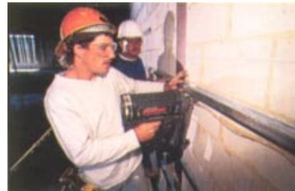
*Rodney Bledsoe fastens wall hatt channel to concrete block.*
