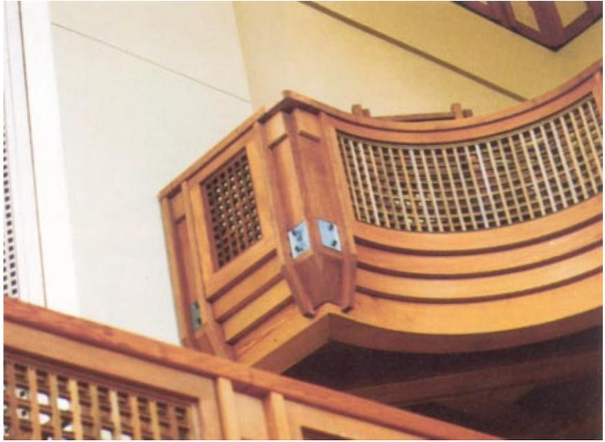
*Amid the mass of timbered elements inside the hall, a synthetic stucco in “Tanglewod Yellow” delicately masks the concrete block. (Photo by Christopher Brown.)*
