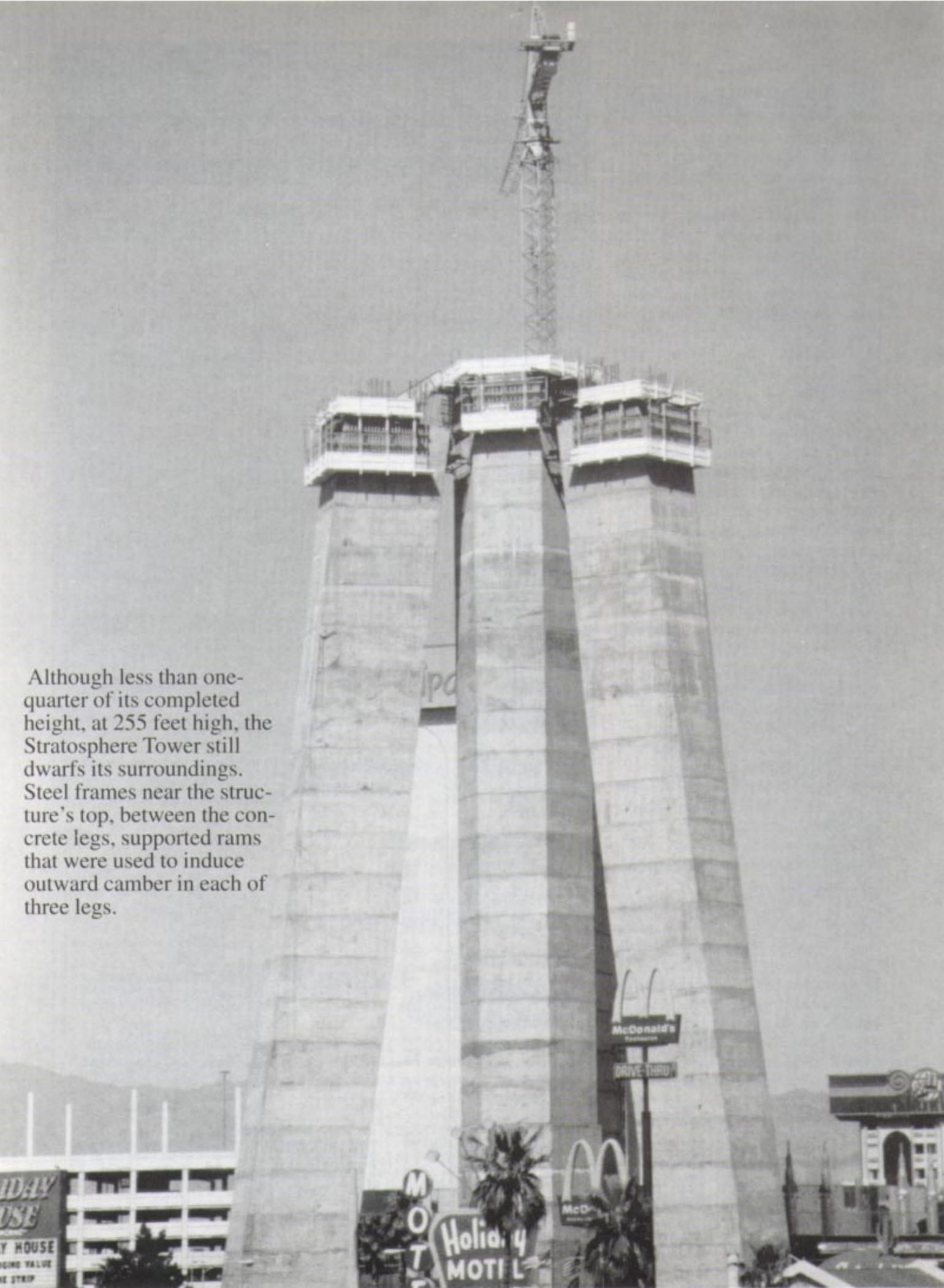
Although less than one-quarter of its completed height, at 255 feet high, the Stratosphere Tower still dwarfs its surroundings. Steel frames near the structure's top, between the concrete legs, supported rams that were used to induce outward camber in each of three legs.
