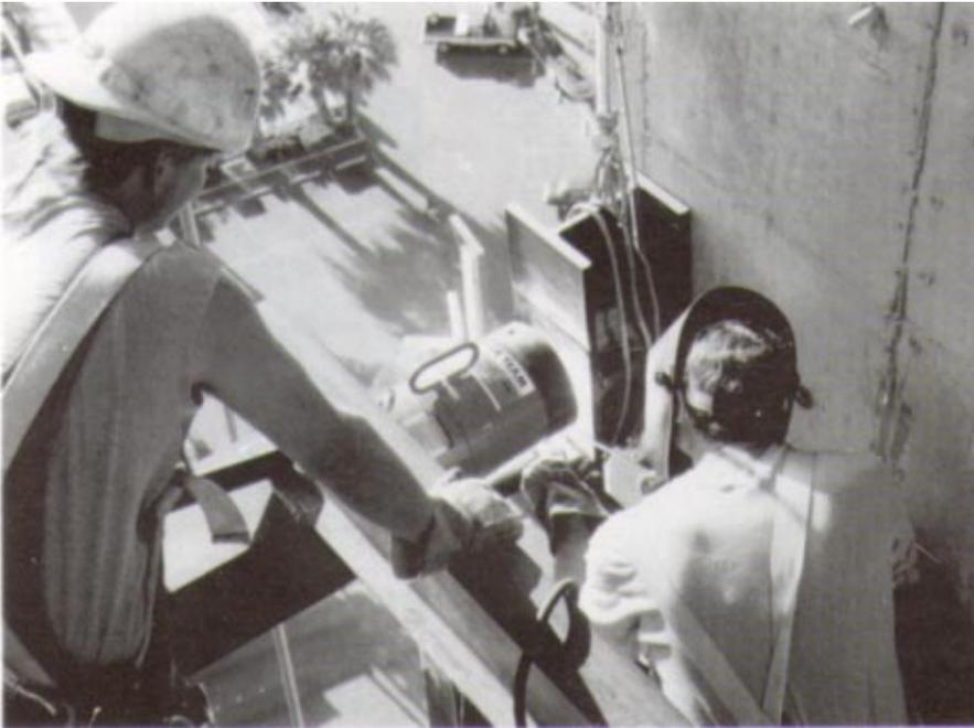
*The Stratosphere's construction workers make final adjustments on the steel frame supporting the rams. The rams' hydraulic force deflected the concrete to induce a camber in each of three concrete legs.*
