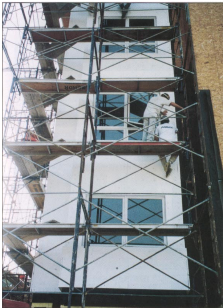
Installation of water-barrier system
