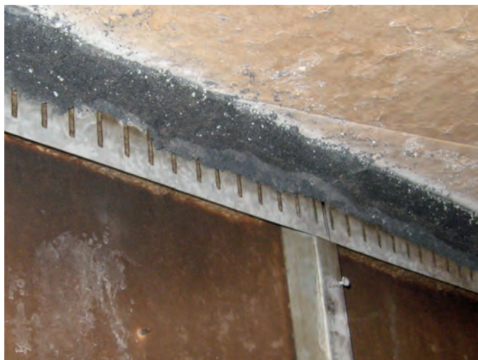
Expanded intumescent strip after fire test
