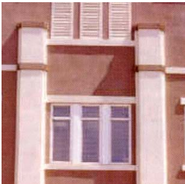
Triangle Plastering Systems used 37 different colored EIF systems on the Southlake Town Square project.
