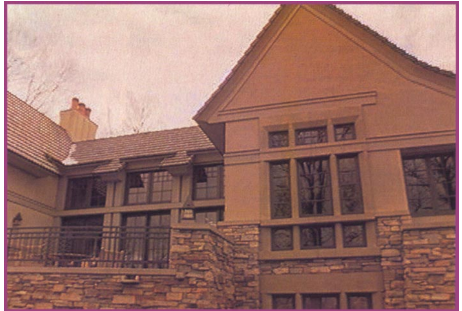
The base coat was applied to the exterior cement board surface.
