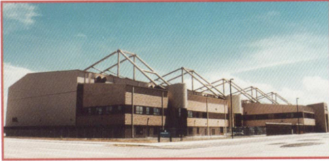
Antisubmarine Warfare Maintenance and Training Facility at the Jacksonville Naval Air Station, Jacksonville, Fla.
