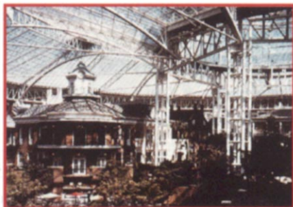
Opryland Hotel, (Phase IV, The Delta), Nashville, Tenn.
