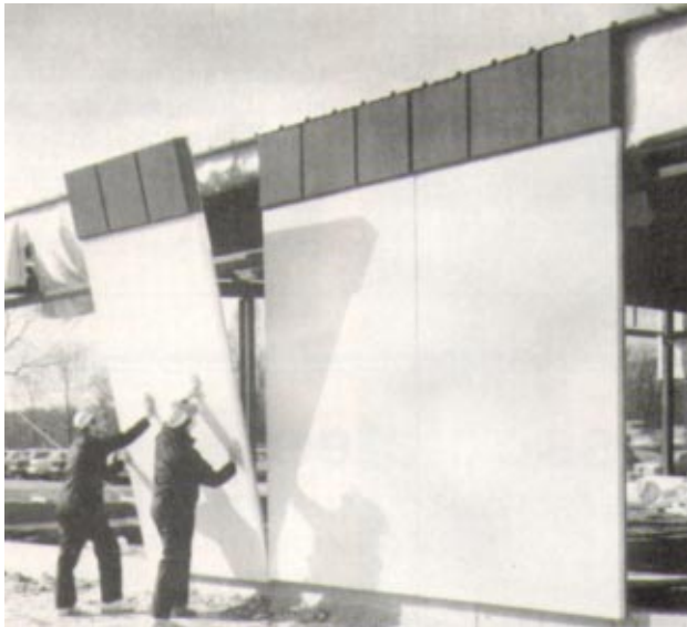
Men positioning Metalite Panel System.
